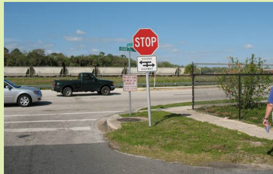
The sign for no left turns during school arrival and dismissal is difficult to see
