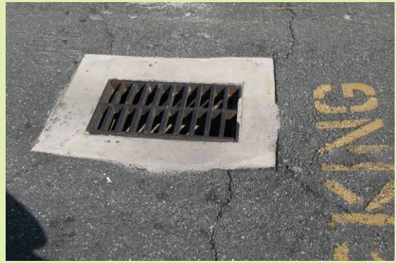
Bicycle tires may catch on this type of drainage grate
