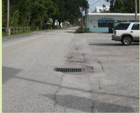
Myrtle Avenue looking north along the east side of the roadway
