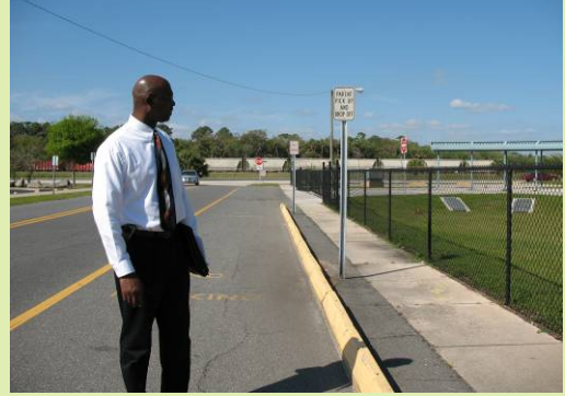
Stephan Harris, MPO Bicycle and Pedestrian Coordinator, examines the free-standing curb that may create a trip hazard
